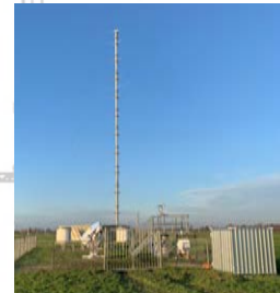
Scanning dual frequency cloud radar and microwave radiometer installed on wind profiler site in Cabauw
