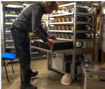
Installation of ICOS Level 1 equipment in Cabauw main building
