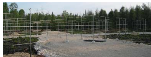
Figure 2. Picture of the Negro Creek radar. This is typical of all the radars in the network.
