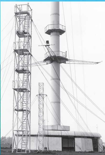
Close to the ground the building below the mast would disturb measurements. Therefore a 10 m and 20 m side mast were erected for observations below 20 m. Photo J.G. van der Vliet, August 1973.
