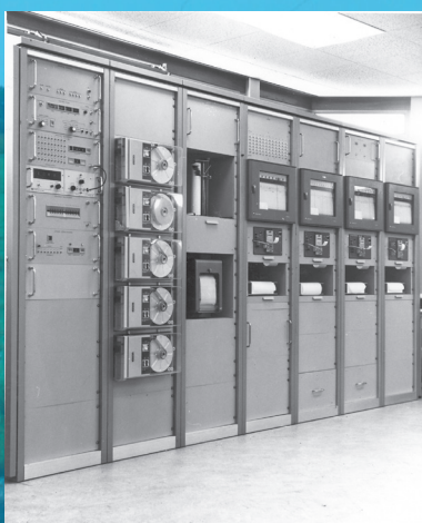
In the pre-digital period data acquisition was realised with paper tape and analogue recorders. Photo J.G. van der Vliet, August 1973.
