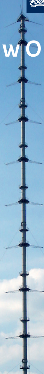
Close to the ground the building below the mast would disturb measurements. Therefore a 10 m and 20 m side mast were erected for observations below 20 m. Photo J.G. van der Vliet, August 1973.
